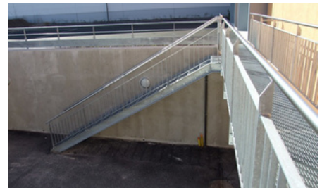
Stairs and canopies
